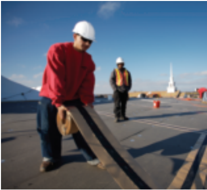
Install QuickSeam R.M.A. Strips.
